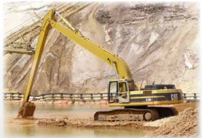
Long reach excavator
